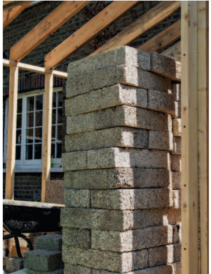
Owing to the unique mechanical properties of hempcrete, blocks still need to be cast around a structural frame.
