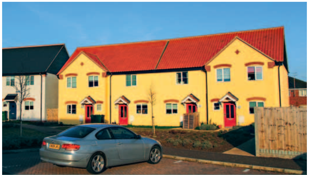
Hempcrete terrace at a housing association development in Diss, in Norfolk, constructed from cast-in-situ hempcrete around a timber frame.
