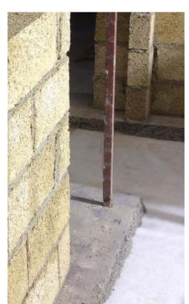
The hempcrete blocks, which are 300 mm thick, are being used in the ground floor walls of the building – a play barn – with a total area of 174 m<sup>2</sup> of blocks being installed. Hempcrete blocks are formed from hemp 'shiv', the chopped woody stem of the industrial hemp plant, combined with a binder of natural hydraulic lime.
